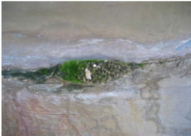
**Cracks on a fiberglass tank**
