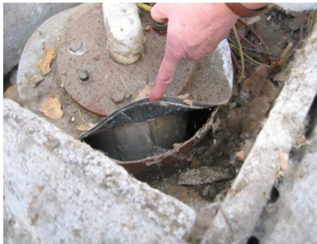
**Seal on wellhead not watertight**
